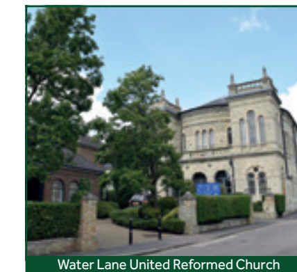
Water Lane United Reformed Church
